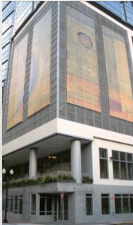
DyneTech Centre Orlando, FL - Fabric Wall Panels
